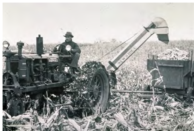
Figure 10. Corn harvest with a tractor-drawn corn picker.
